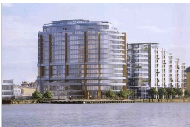
Bridges Wharf, Battersea
